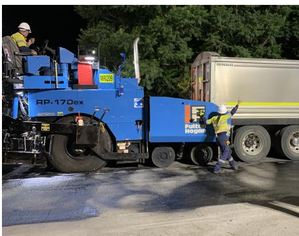
a) Truck positioning to commence paving CRM OGA
