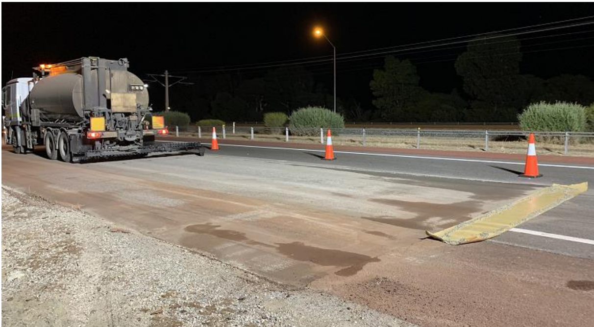
Figure 5.6: Spray truck positioning to spray on L2, SLK 25.46, Kwinana Freeway
