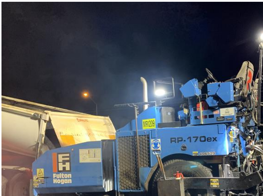
Figure 5.10: Visible fuming when truck loads paver with CRM OGA (alternative PSD) on Kwinana Freeway
