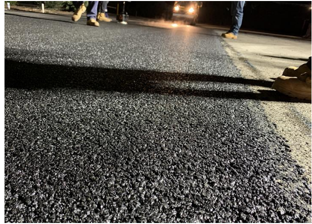
d) Compacted section of CRM OGA
