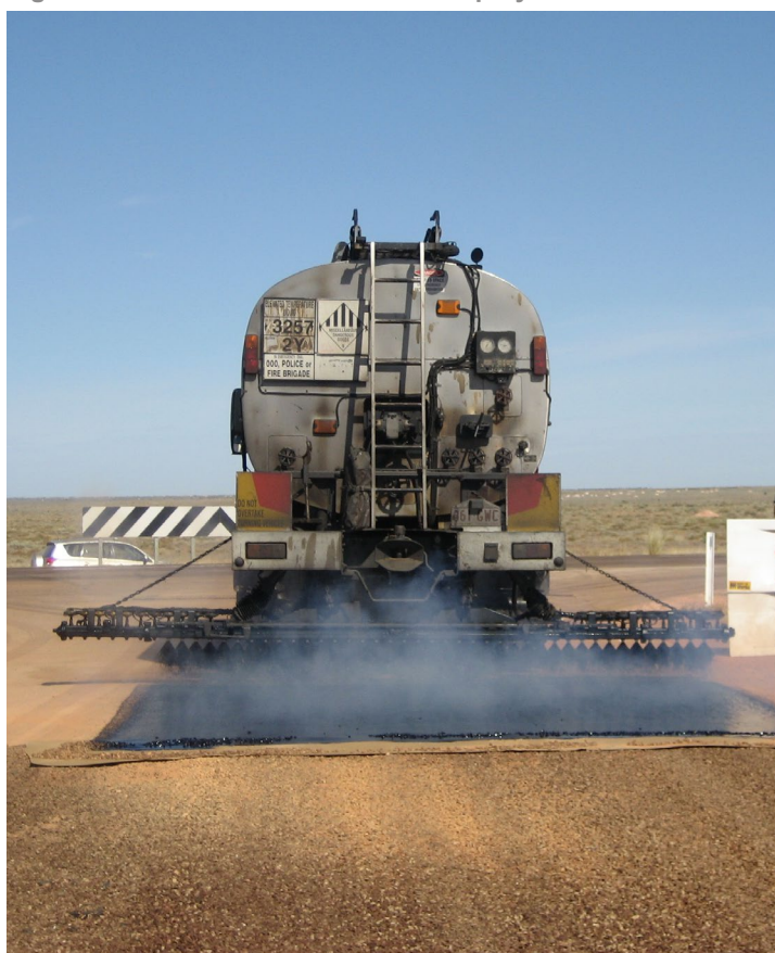
Figure 1: Crumb rubber bitumen sprayed onsite
