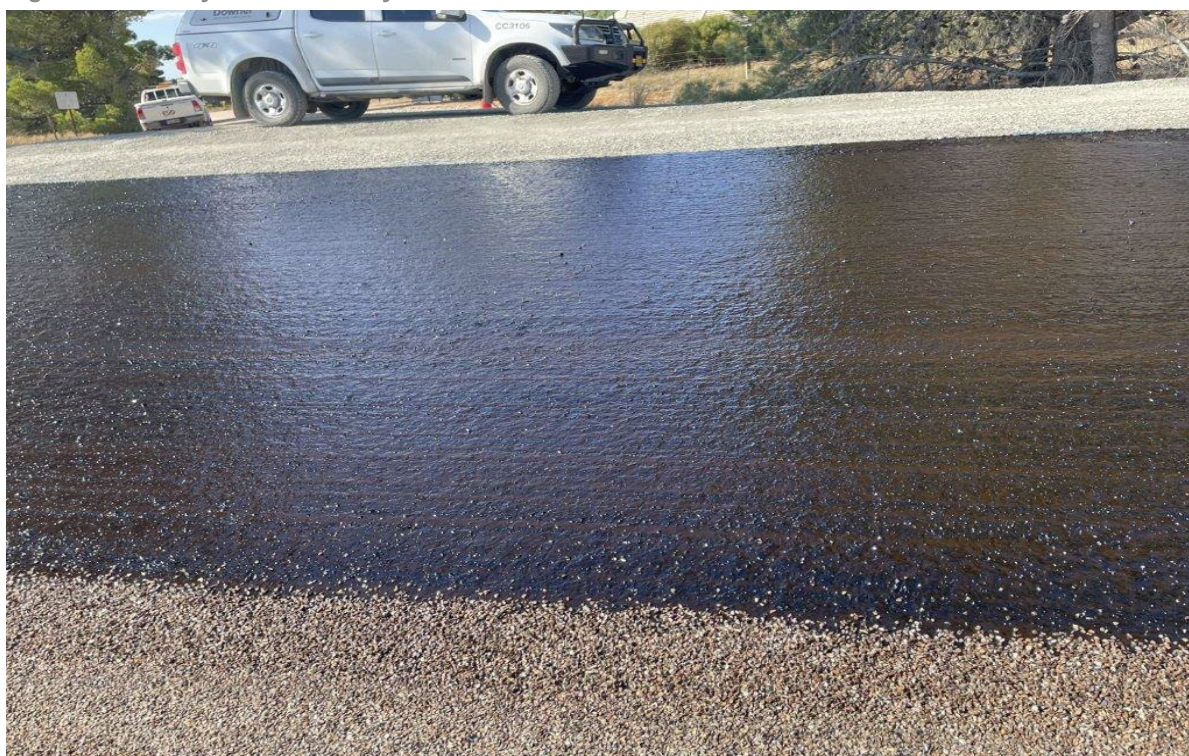
Figure 3: Recently sealed laneway
