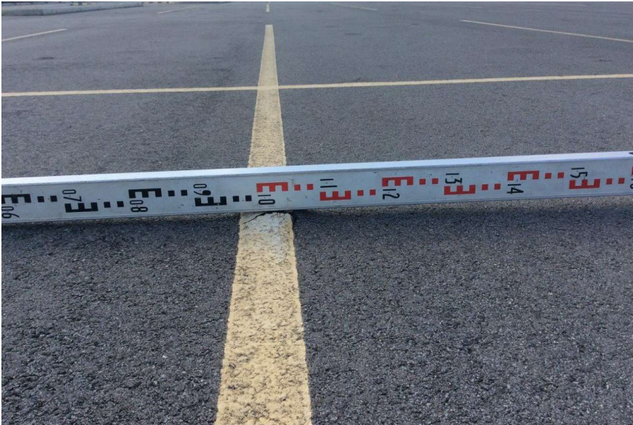
Figure 7.2: Example of surface blistering within a public car park
