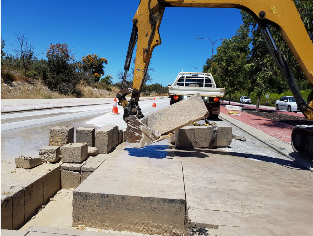
Figure 4.9: Warton Road CRC basecourse sampling
