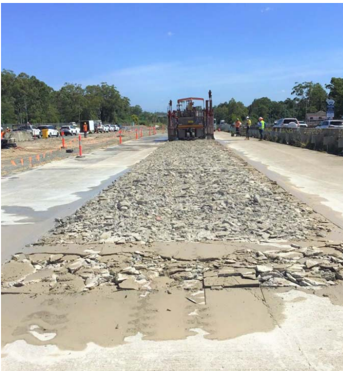
Figure 4.13: Rubblisation works
