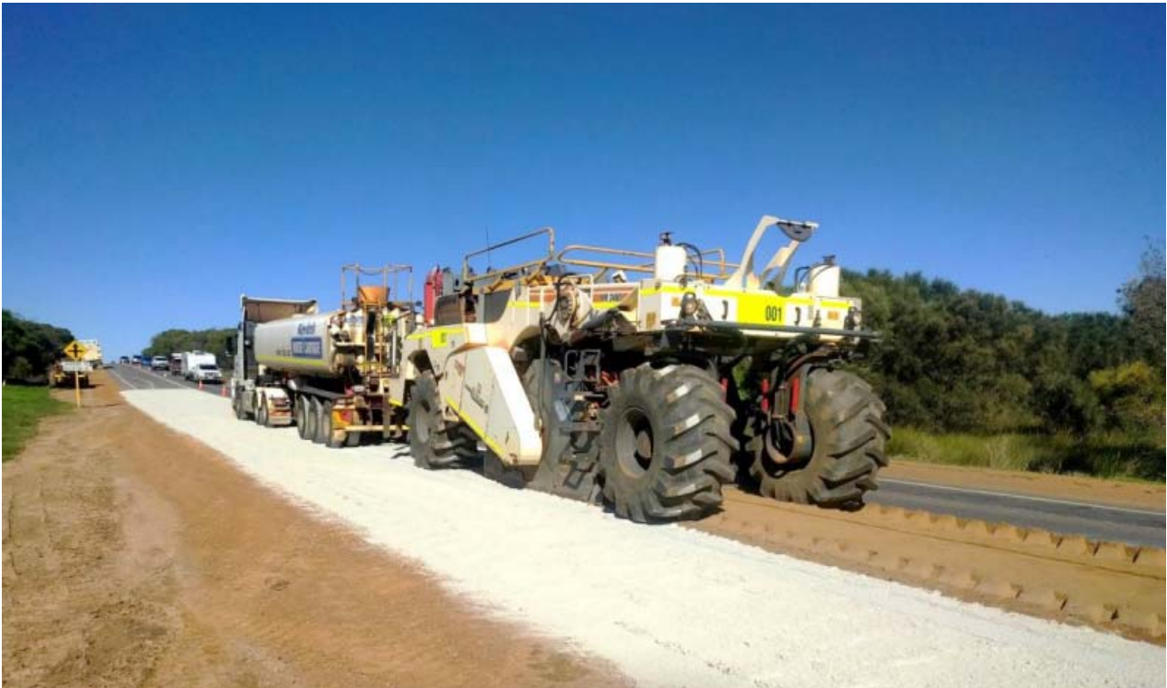
Figure 4.10: Cementitious stabilisation construction
