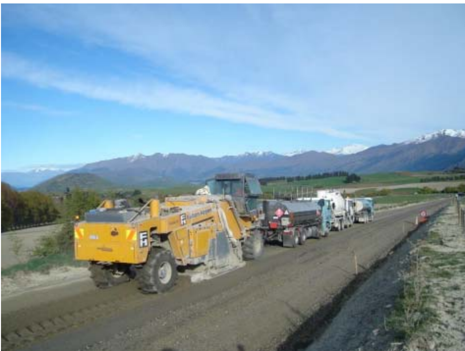
Figure 4.9: Foamed bitumen stabilisation construction train
