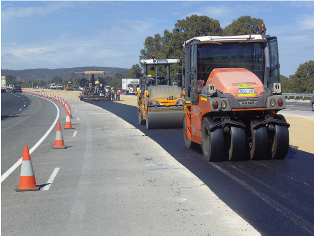
Material compaction during paving operation at Perth trial site
