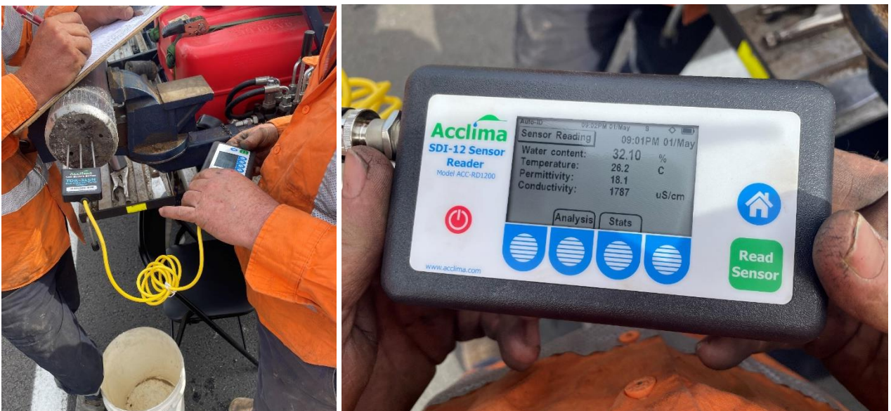
Figure 3.12 On site measurements of temperature and moisture content
