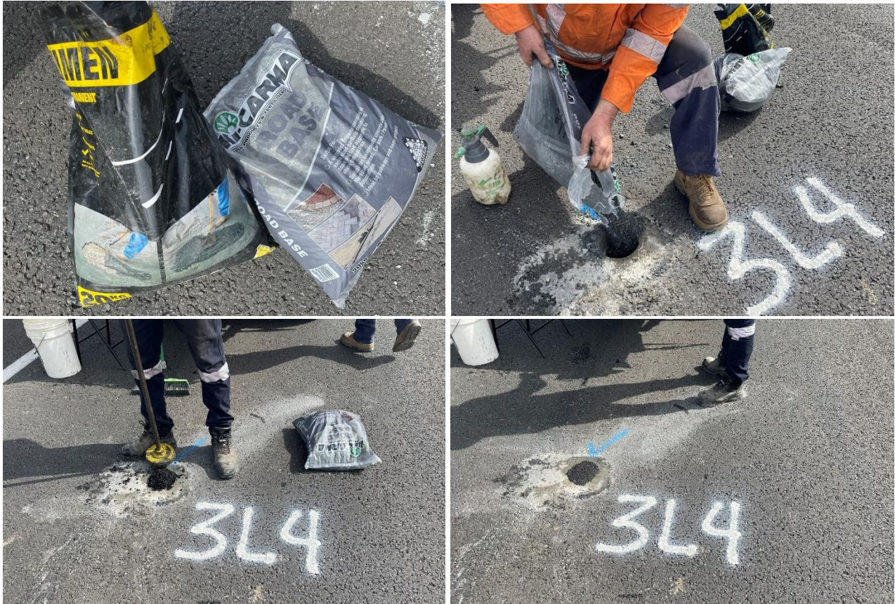
Figure 3.13 Reinstating using certified road base and cold mix AC
