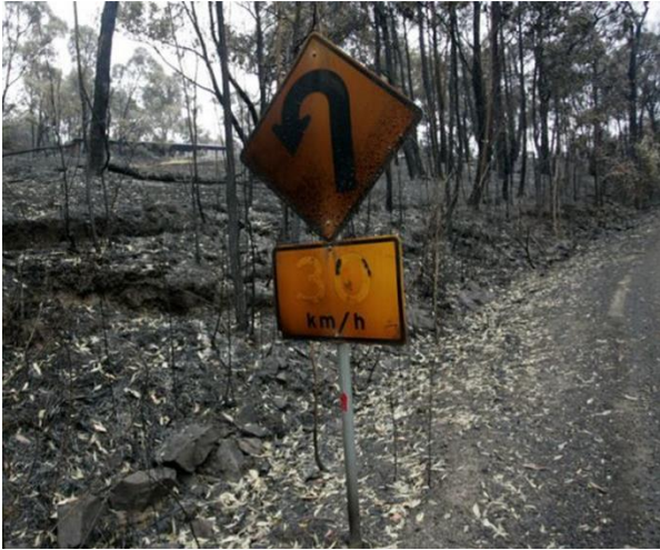
Figure 2.9: Bushfire damage to safety infrastructure
