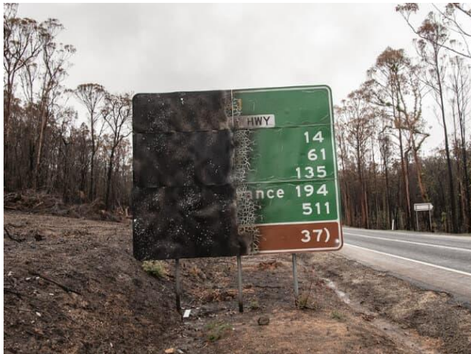
Figure 2.10: Bushfire damage to road signs
