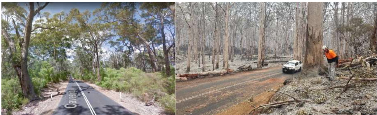
Figure 4.11: Bushfire damage to roadsides
