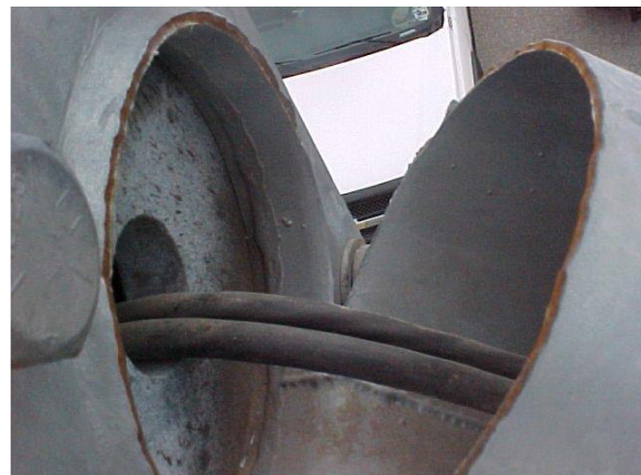
b. Fatigue failure at mast-arm connection
