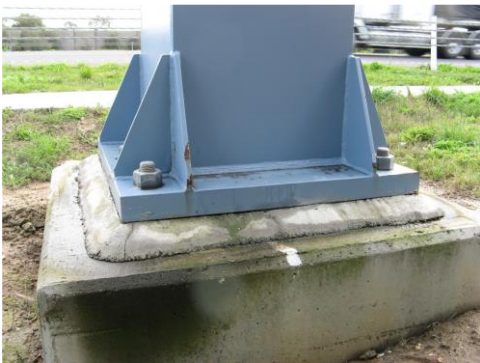
Figure 2.6: Base plate anchorage assembly
