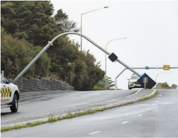
Figure 2.8: Failure of a cantilever sign structure in Auckland, NZ, 2019
