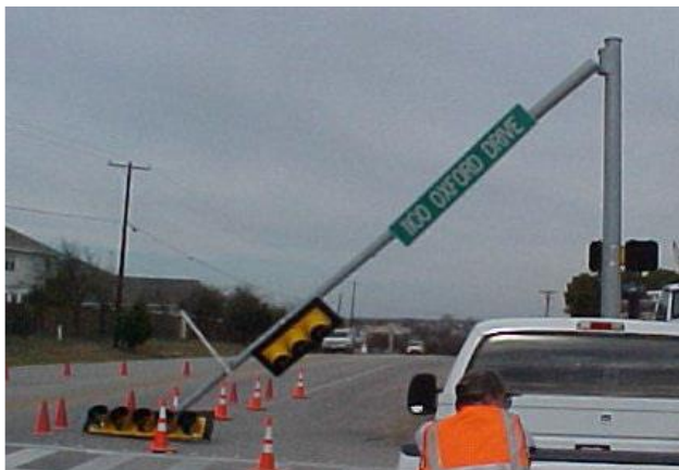
a. Fallen cantilevered arm
