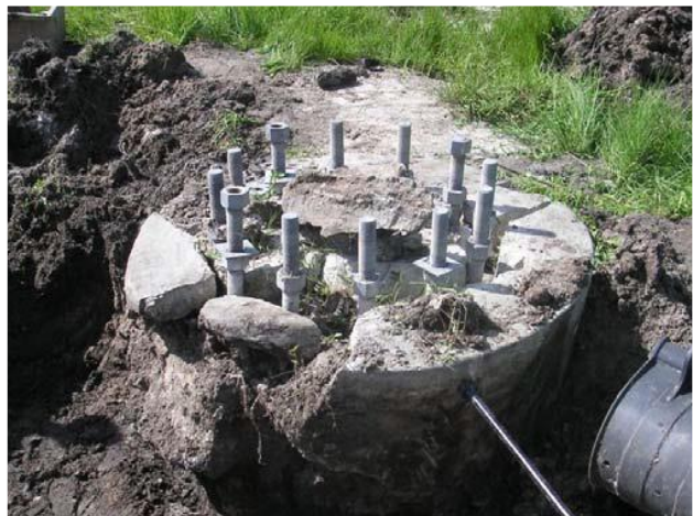
b. Close-up of foundation concrete breakout
