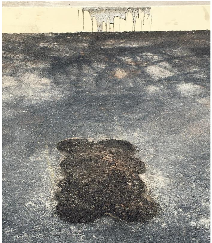
Figure A 13: Cold-mix backfill
