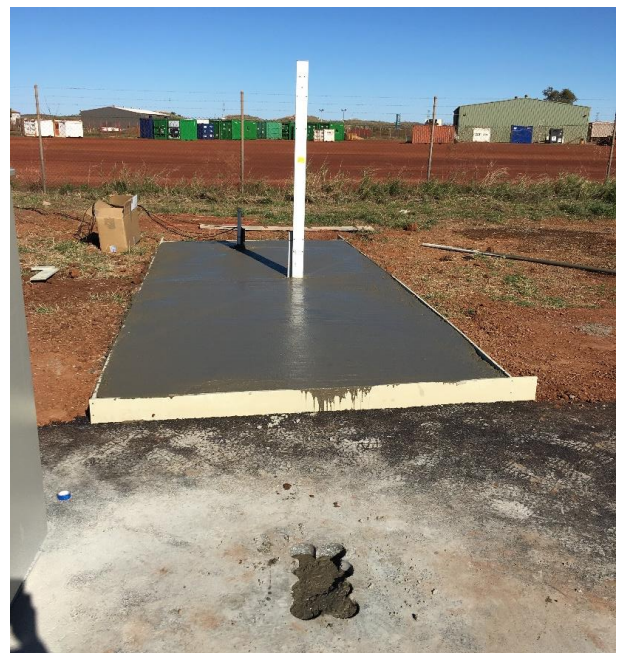
Figure A 15: Concrete base and back fill
