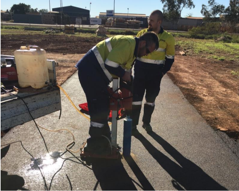
Figure A 3: Coring
