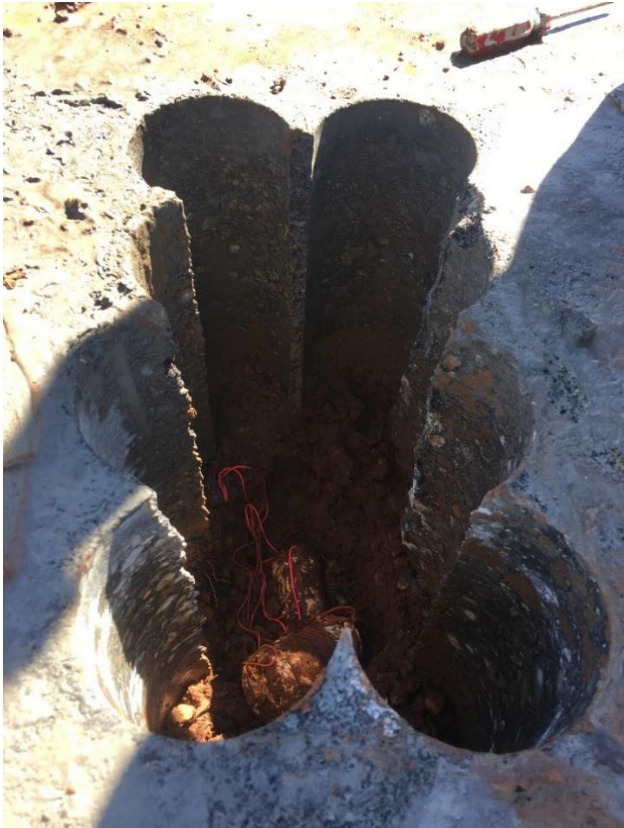
Figure A 5: Cored section of pavement
