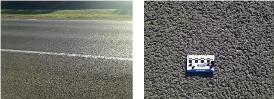
Figure 4.6: Roe Hwy, southbound carriageway, North of Helena Valley Rd overpass
