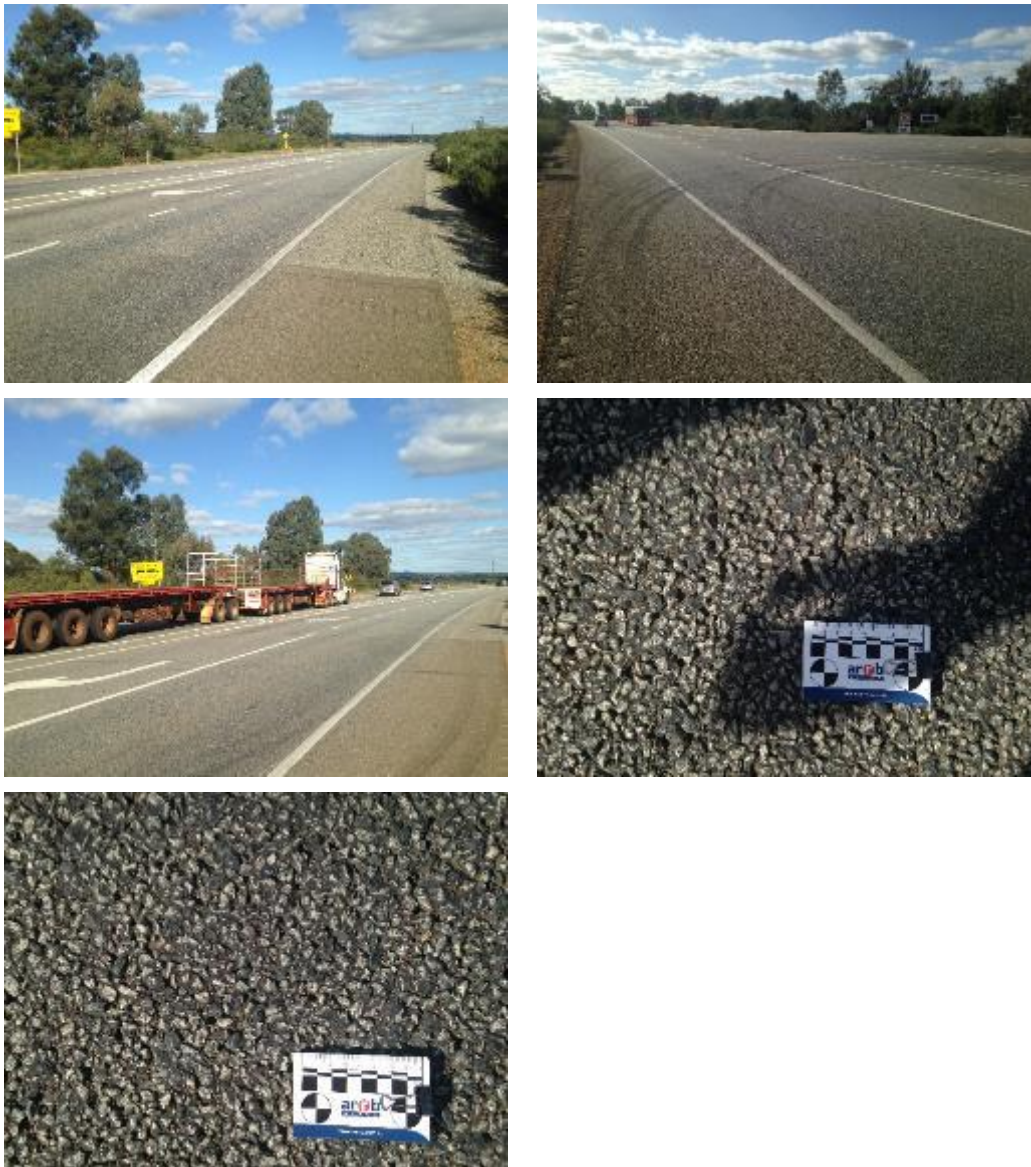
Figure 4.13: Great Northern Hwy, Wandena Rd intersection (SLK 32.72)
