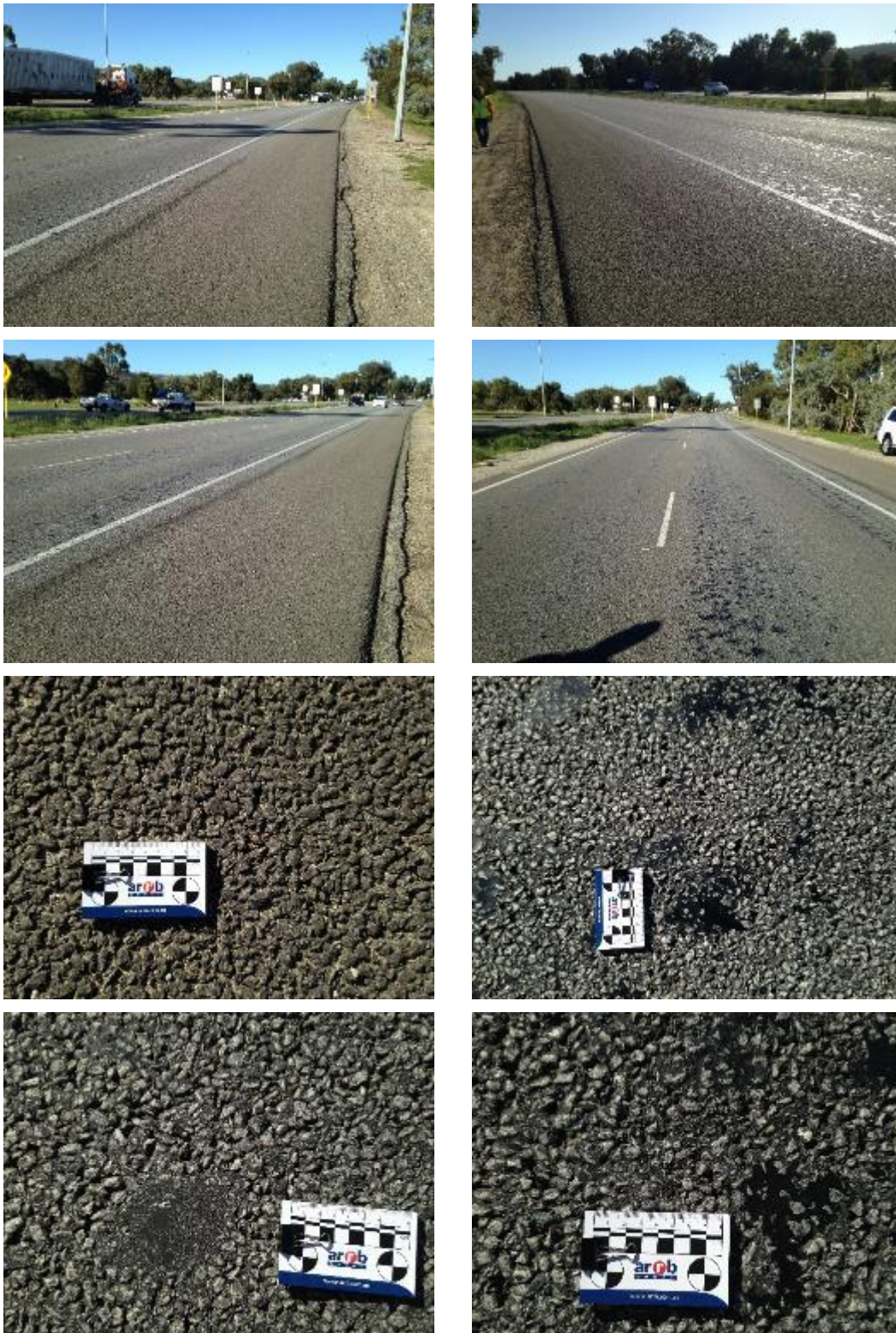
Figure 4.1: Tonkin Hwy, northbound carriageway, Gosnells Rd East – Kelvin Rd (SLK 23.49 – 24.13)
