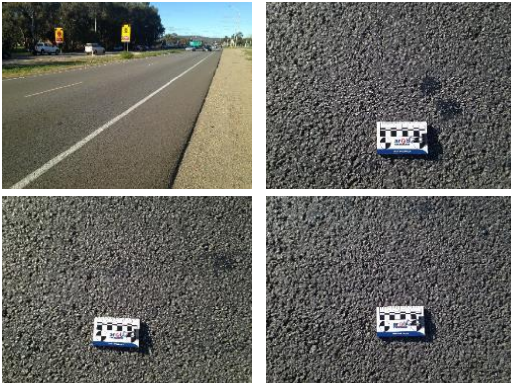
Figure 4.15: Great Eastern Hwy Bypass, eastbound carriageway, Stirling Cres – Abernethy Rd
