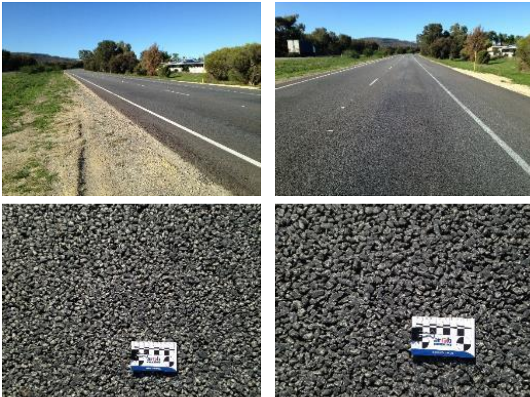
Figure 4.3: Tonkin Hwy, northbound carriageway, Gosnells Rd East – Kelvin Rd (SLK 22.99 – 23.49)
