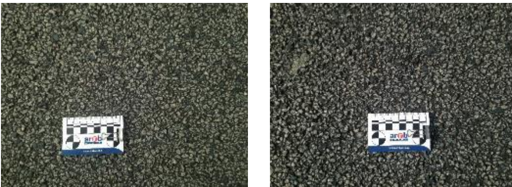
Figure 4.10: Wanneroo Rd, northbound carriageway, Tadorna Ent – Ashley Rd
