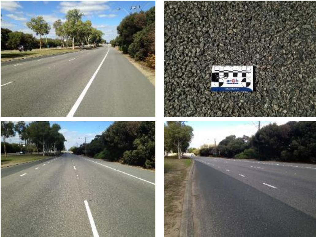
Figure 4.9: Marmion Ave, northbound carriageway, Readshaw Rd – Seacrest Dr
