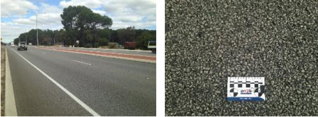
Figure 4.11: Wanneroo Rd, southbound carriageway, Tadorna Ent – Ashley Rd
