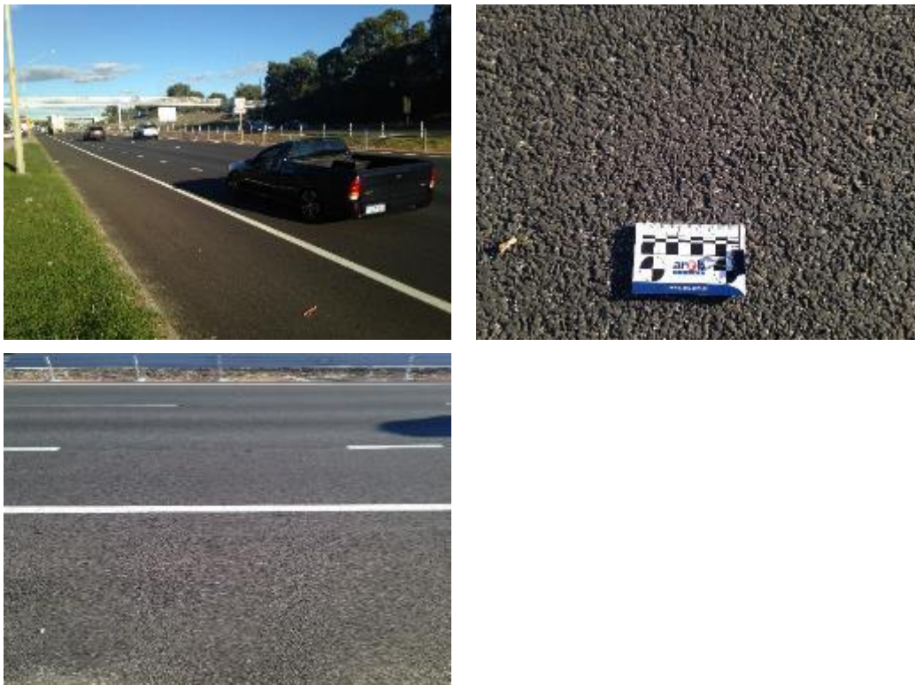
Figure 4.4: Tonkin Hwy, next to Great Eastern Hwy southbound on-ramp
