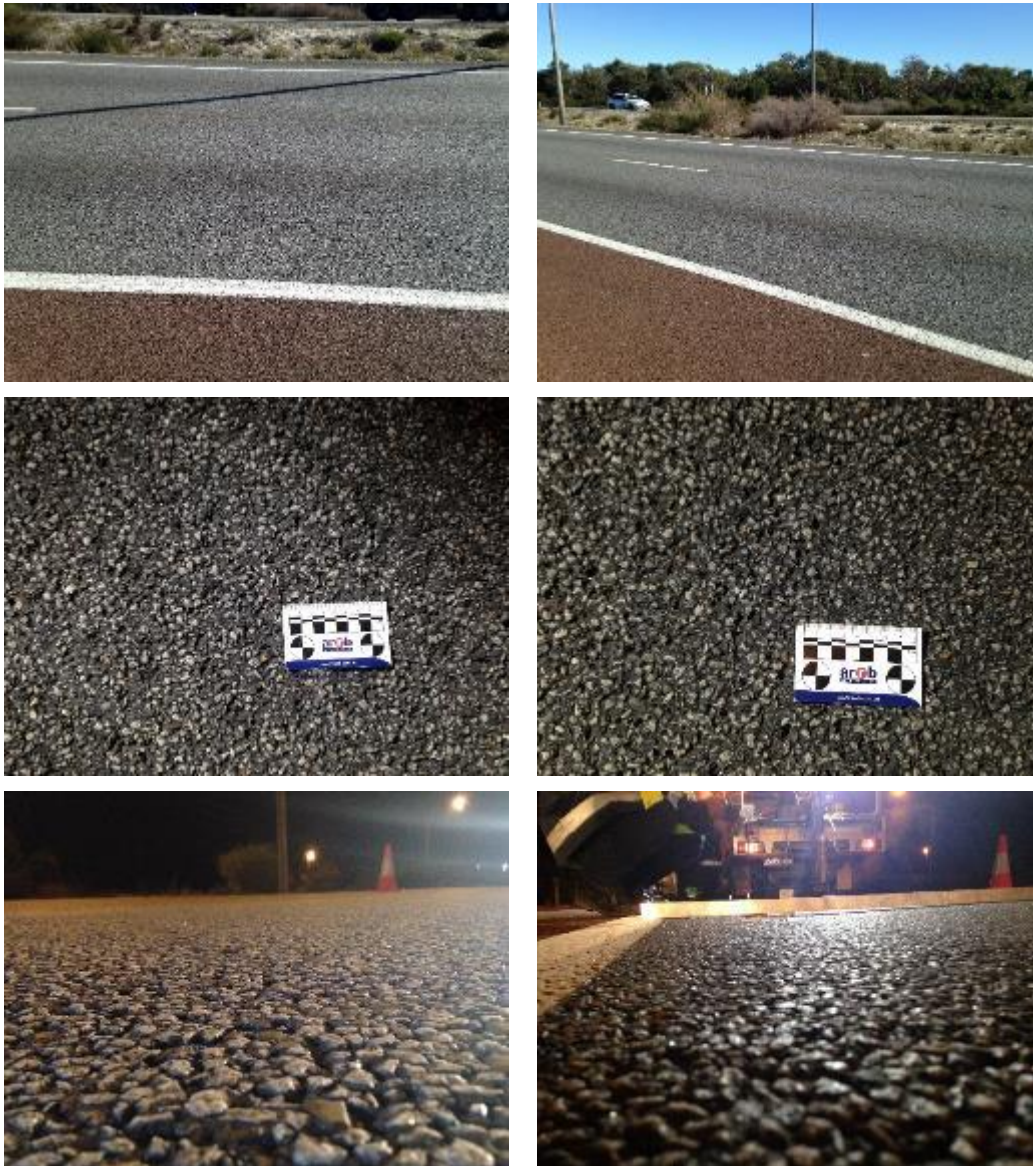
Figure 4.5: Roe Hwy, westbound carriageway, South St – Karel Ave
