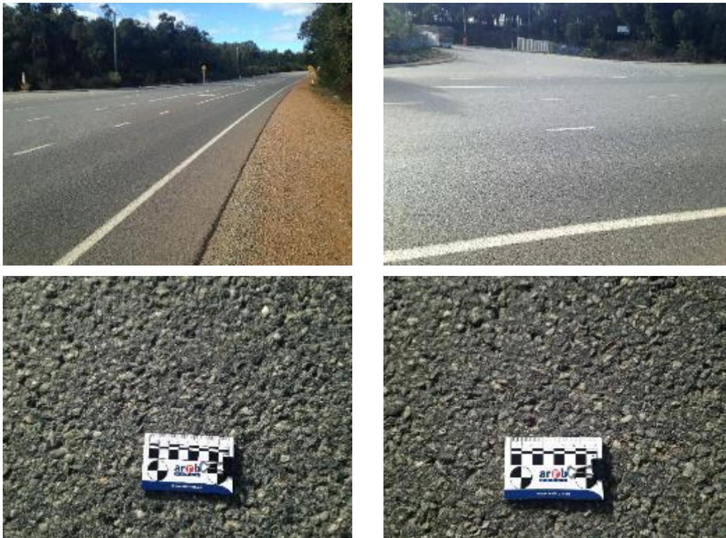
Figure 4.14: Toodyay Rd, westbound lane, quarry entrance
