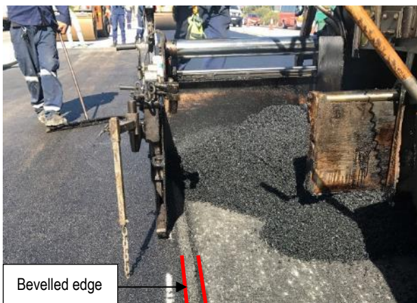
Figure 7.16: Joint overlapping from paver
