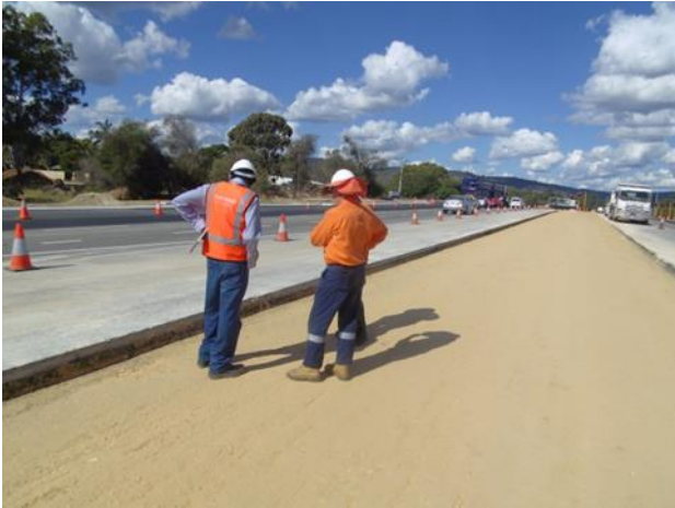
Figure 5.6: Visual inspection of subbase
