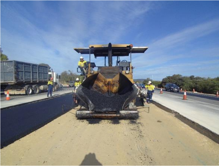
Figure 7.7: Paving of Layer 1 of LR1
