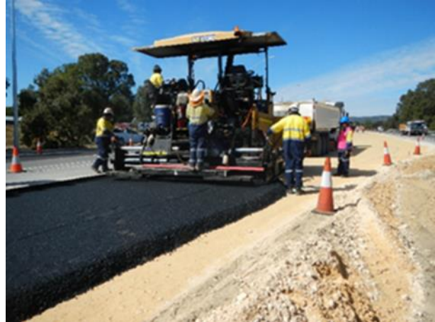
Figure 7.4: Paver operation
