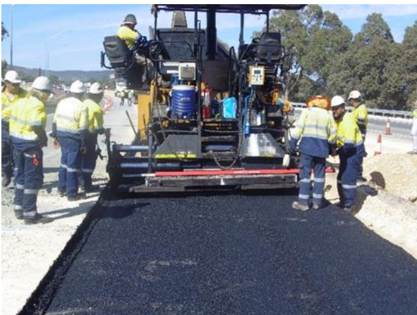
Figure 7.5: Paving operation southbound
