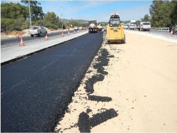
Figure 7.14: Cut edge with excess material
