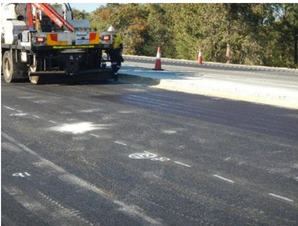
Figure 7.8: Application of tack coat
