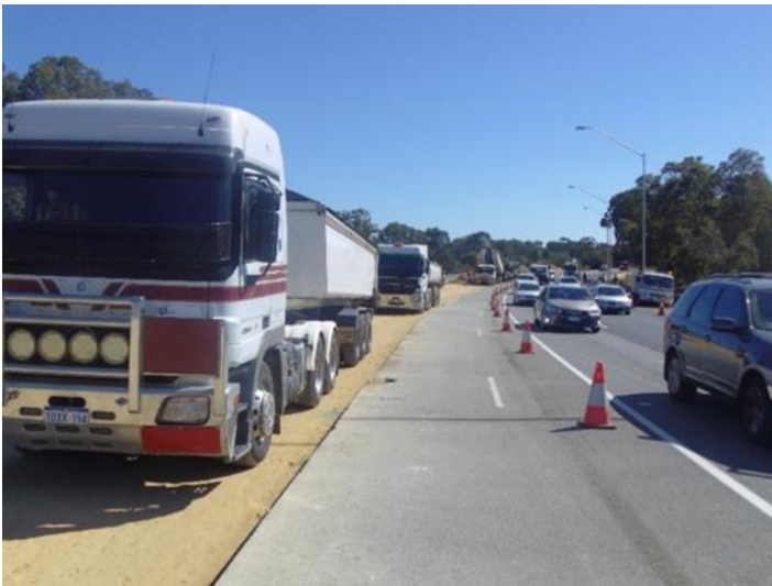
Figure 7.1: EME2 asphalt being delivered
