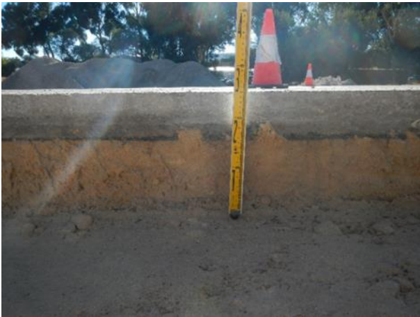
Figure 5.4: Thickness of subbase
