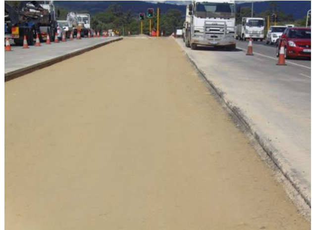
Figure 5.7: Subbase ready for asphalt placement
