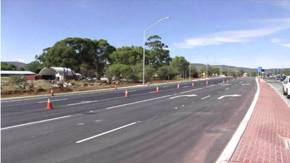
Figure 7.39: Finished wearing course and line marking
