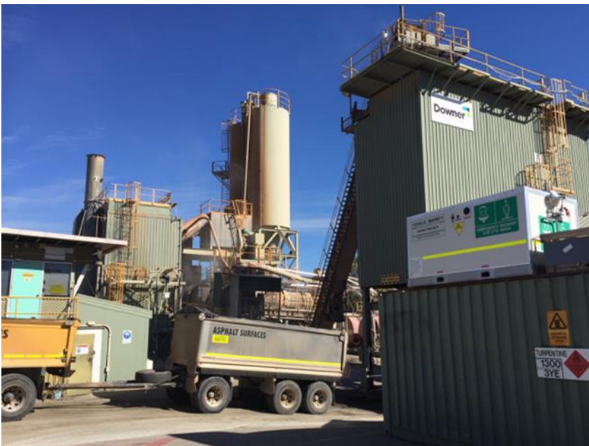
Figure 6.2: Downer Group plant used for the trial
