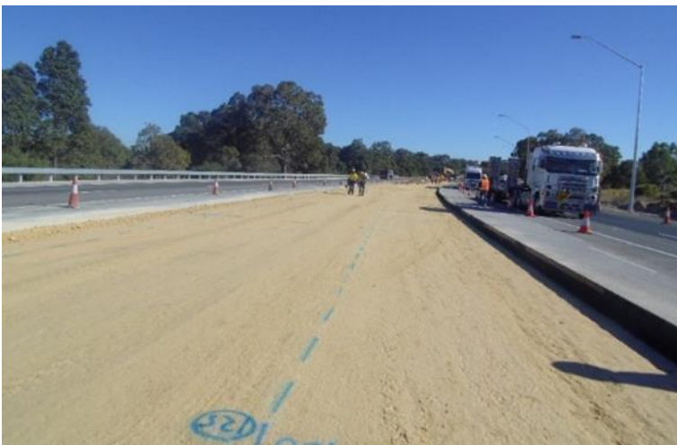
Figure 7.2: Limestone subbase marked ready for EME2 mix placement
