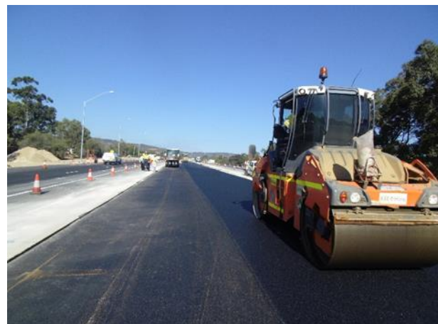
Figure 7.13: Static rolling to finish
