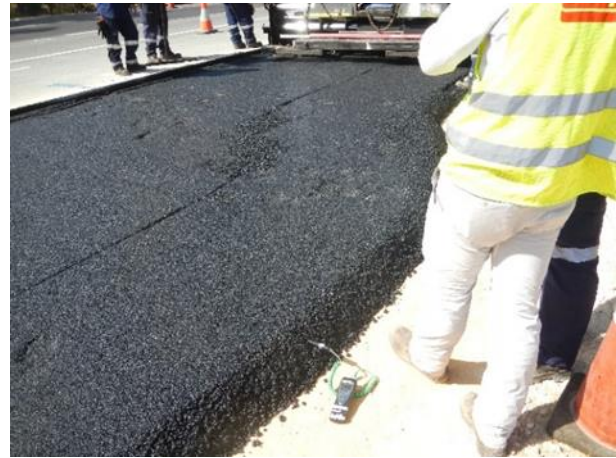
Figure 7.19: Mat compactor with digital thermometer
