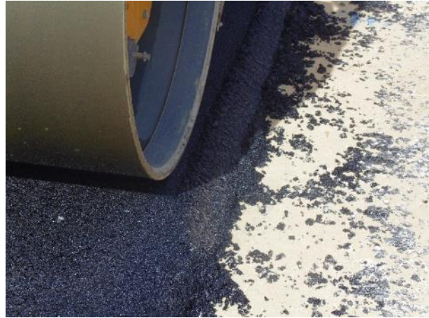
Figure 7.15: Roller pressing pavement edge
