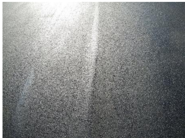
Figure 7.17: Finished Layer 2 joint
