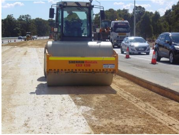
Figure 5.3: Vibrating smooth drum roller
