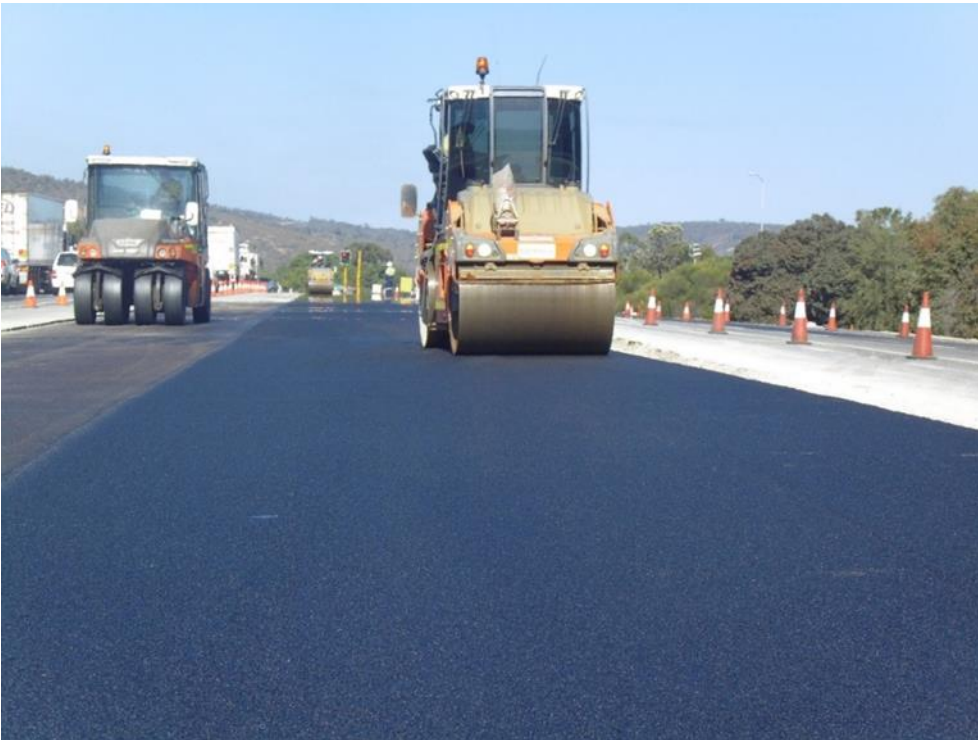
Figure 7.36: Surface appearance after compaction
