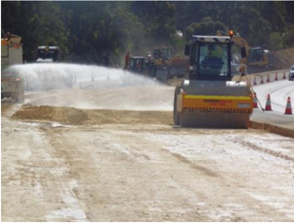
Figure 5.2: Construction of subbase
