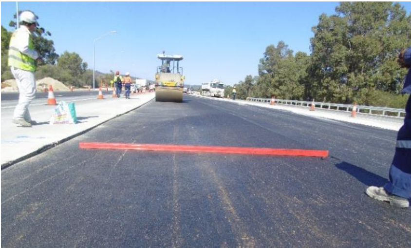
Figure 8.23: Checking shape in a transverse direction using 3 m straight edge
