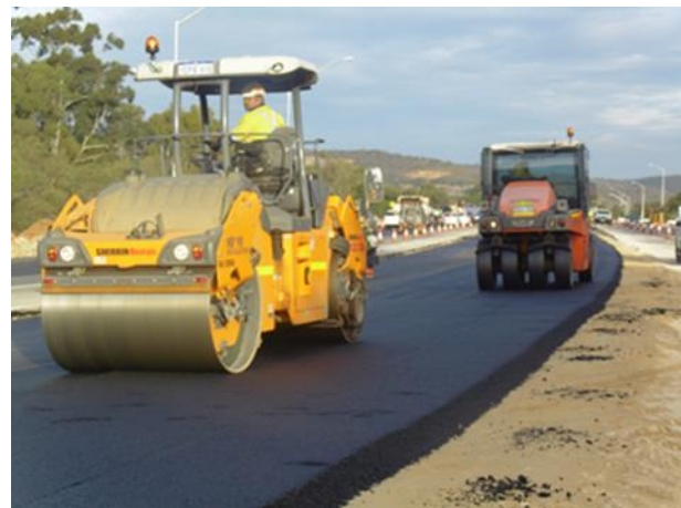
Figure 7.11: Multi tyred roller behind the vibrating roller
