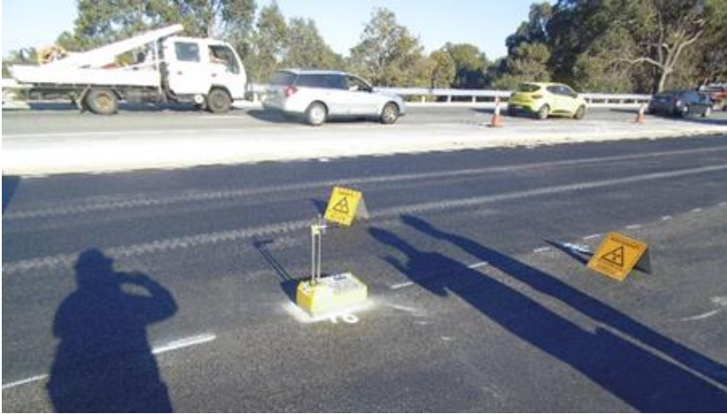
Figure 8.14: Nuclear gauge densities recorded in the joint lines
