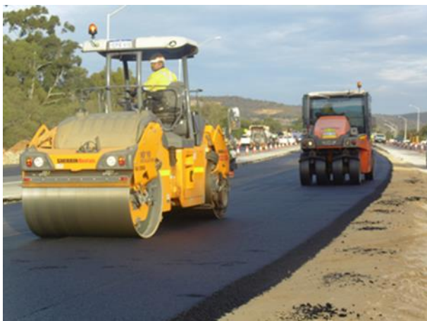
Figure 7.12: Multi-tyred roller behind the vibrating roller
