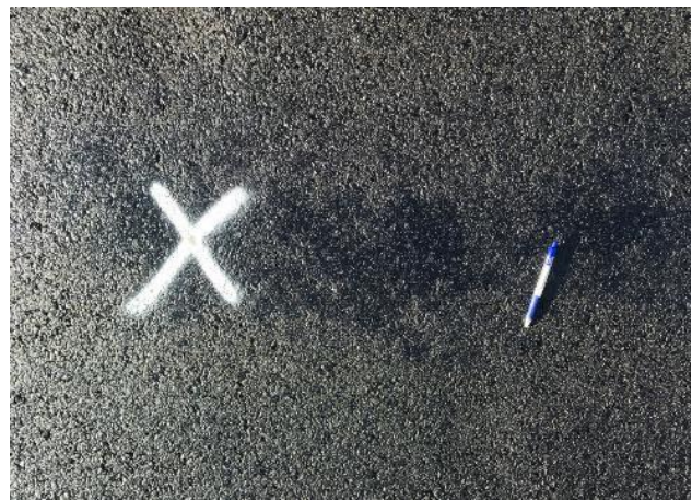
Figure 7.38: Surface flush patches
