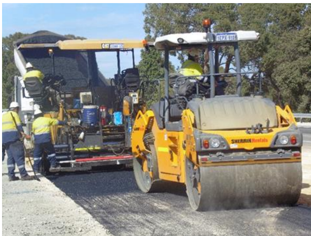
Figure 7.10: Vibrating smooth drum roller
