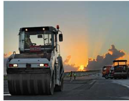
Roland Garros Airport- Expansion of runways and taxiway http://www.nouvelroutedulittoral.re/ 2013
