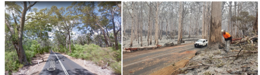
Figure 4.11: Bushfire damage to roadsides
