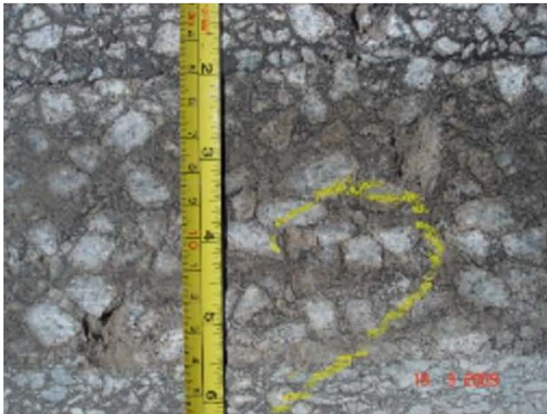
Photo 1: Pavement with three layers of asphalt approximately 200 mm thick.
