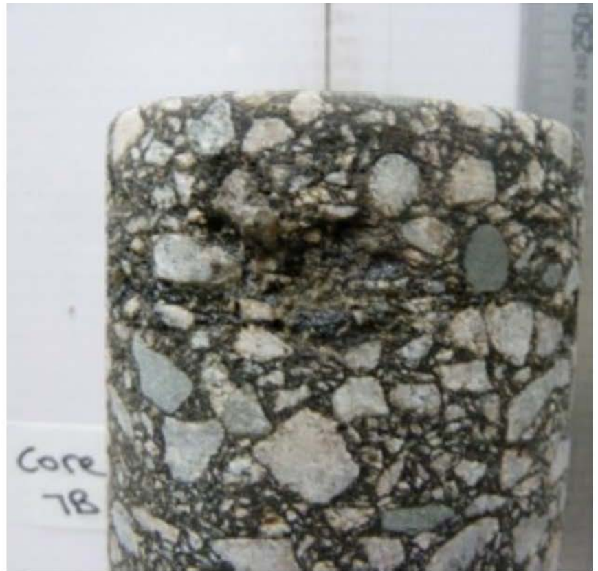
Photo 2: Stripping leading to voided section in core
