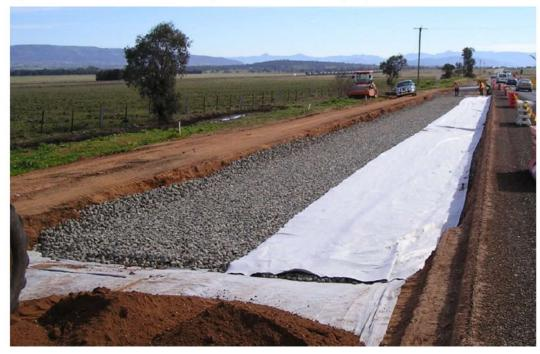
Figure 4.10: Geotextile as separation layer above and below drainage layer
