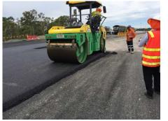
EME2 was developed in France and industry experts came to assist our research into this heavy duty pavement material in Western Australia. Using a strong, durable material that can handle heavy loads with a reduced thickness provides dual benefits of material savings and time savings. Initial trials again provided many learning's and has provided an interim specification.
