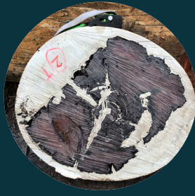
Advanced Epoxy Timber Pile Repair
