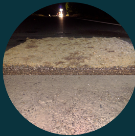
Hydrated Cement Treated Crushed Rock - Base Trial Sections
