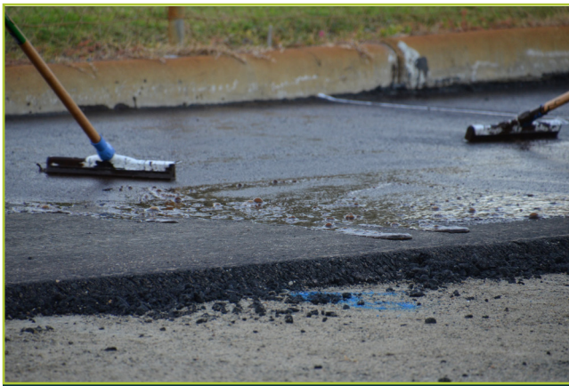
Application of an asphalt bond agent on a test pad.
