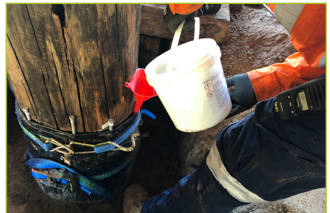
Pouring epoxy into an existing timber pile.
