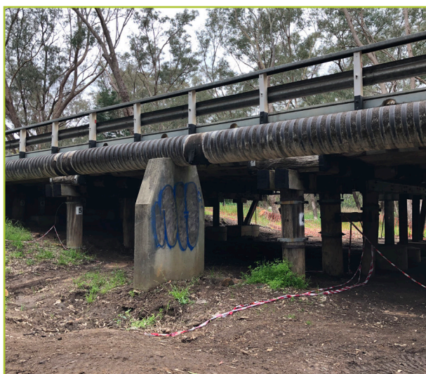
Local bridge with timber piles.
