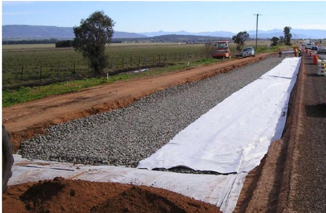
Figure 5.4: Placement of granular material
