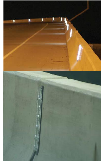
Figure 2.26: LED (only) applications for horizontal alignments (Texarkana, Texas)
