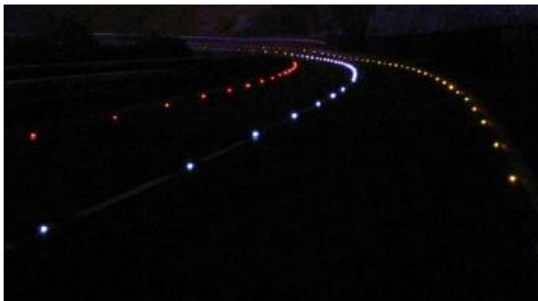
Figure 2.14: Clearview hybrid retroreflective/solar road stud on rural road
