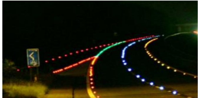
Figure 2.15: Clearview hybrid retroreflective/solar road stud on urban road
