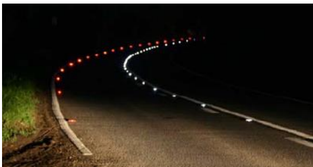
Figure 2.18: On-road hybrid retroreflective/solar road stud on rural road
