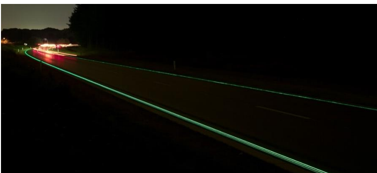
Figure 2.4: Heijmans Glowing Lines, Netherlands trial: demonstrating illumination around a curve
