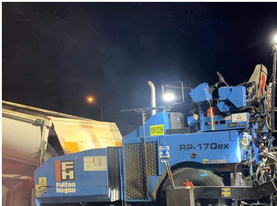
Figure 5.10: Visible fuming when truck loads paver with CRM OGA (alternative PSD) on Kwinana Freeway
