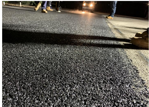
d) Compacted section of CRM OGA
