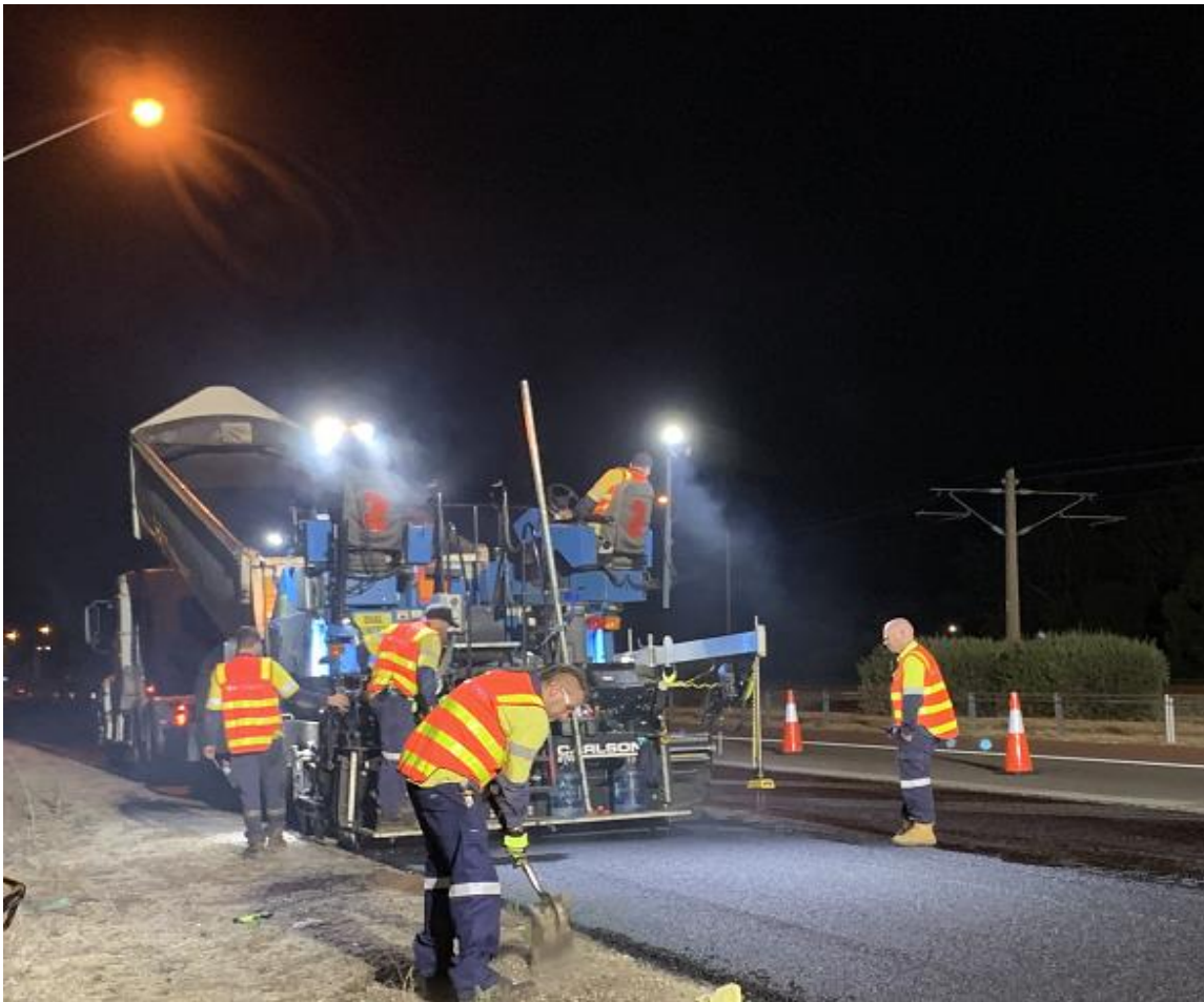
Figure 6.1: Visible fuming with load of mix tipped into paver (1 st truck on site)
