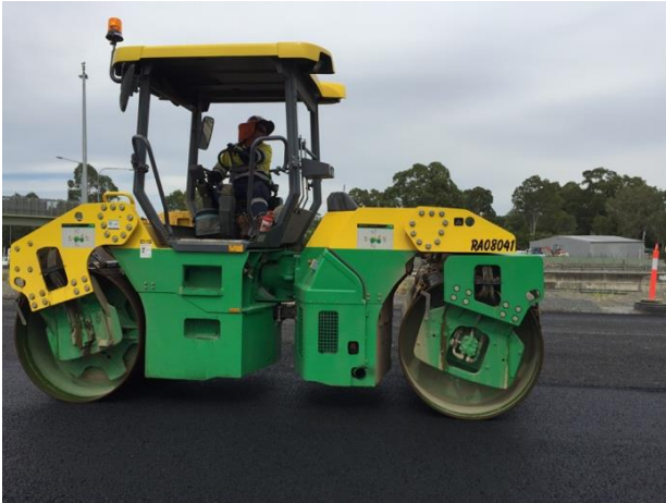
Figure 5.4: Back rolling using 7.7 t steel drum roller
