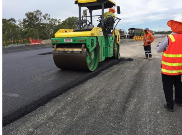
Figure 5.3: Steel drum roller sitting 150 mm from edge
