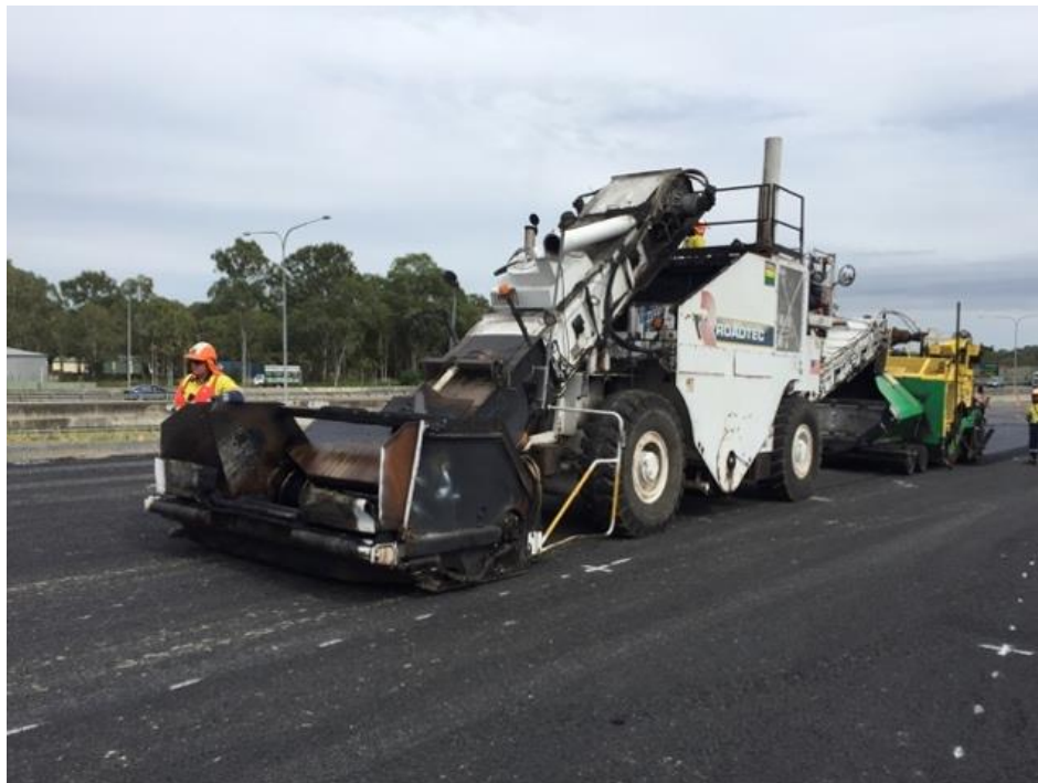
Figure 5.1: MTV during paving operation
