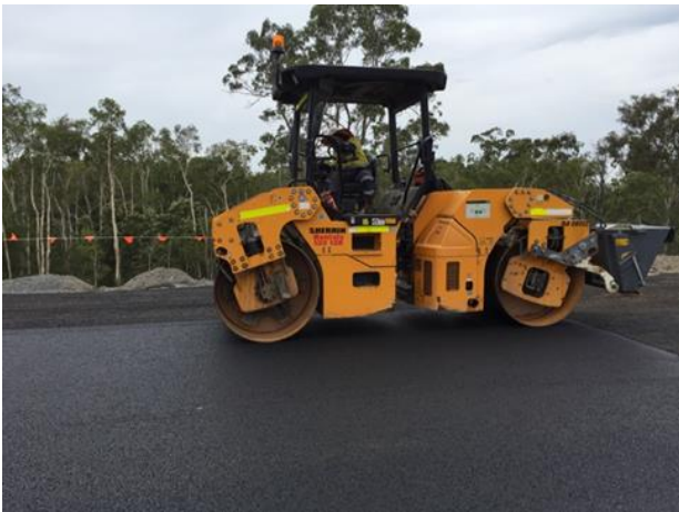
Figure 5.4: Back rolling using 7.7 t steel drum roller
