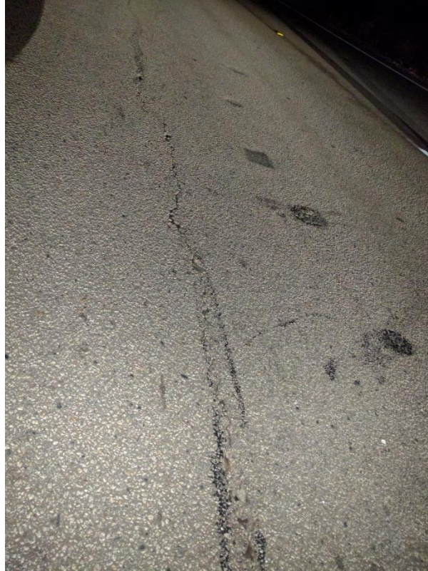
Figure B 6: Thin longitudinal crack in R2 OWP westbound
