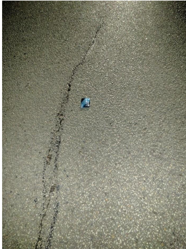
Figure B 6: Thin longitudinal crack in R2 OWP westbound
