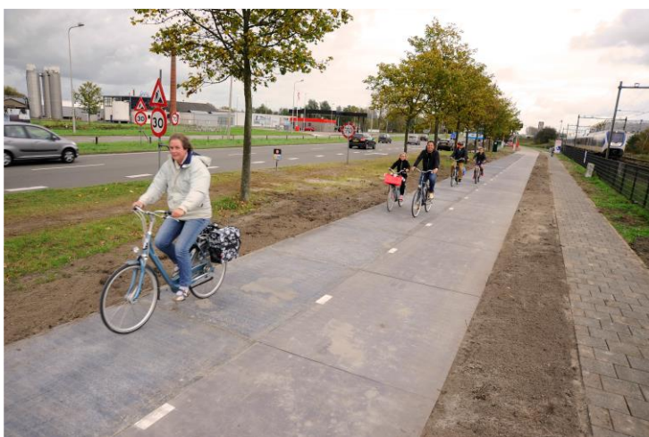
Figure 2.2: SolaRoad bicycle path in Krommenie, North Holland
